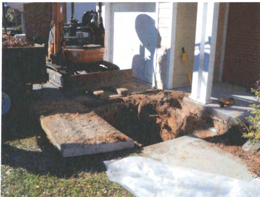
Picture 2: UST 370Aspen excavation .
